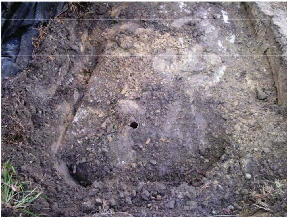
Picture 2: UST 433 Elderberry excavation in progress.
